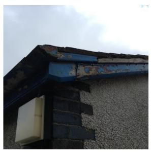
BARGE BOARDS AND VERGES. Rotten Barge Boards and Missing Verge.
